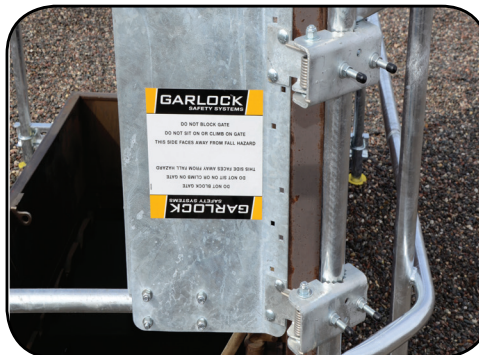
Rugged hinges allow gate tension adjustment.
