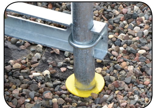
Rail pads protect roof surface.
