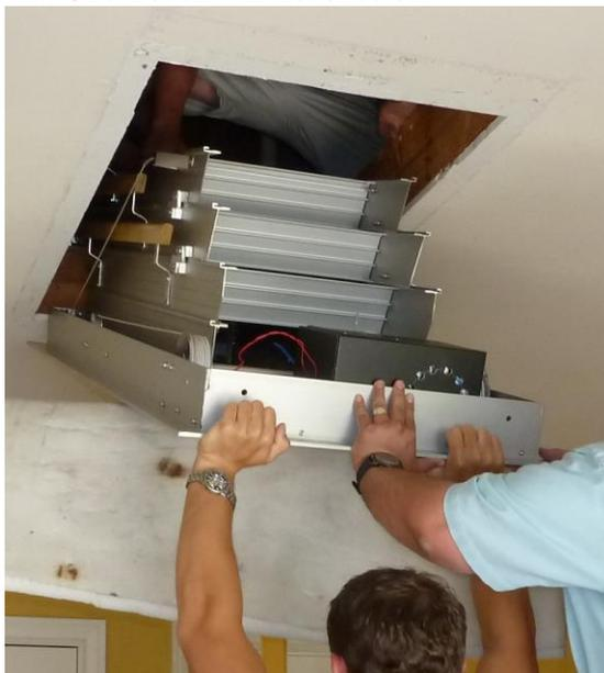
5. Once the overhanging portion of One-Touch is inserted into the opening, the operator of the tool can continue to raise One-Touch until its supporting structure is resting against the ceiling.
