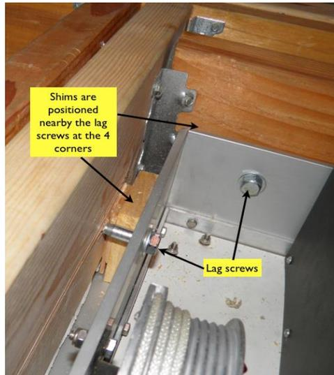
8. One-Touch is now permanently attached to the ceiling support structure.
