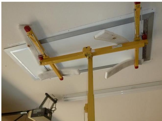
6. One-Touch is now temporarily supported. This is only for temporary support and **NOBODY SHOULD STAND** on One-Touch at this point of the installation.
