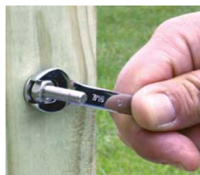
Step 1 Tighten nut to tension
