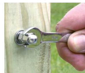
Step 3 Install acorn nut
