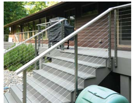
HandiSwage™ Spectrum (p.18) 1-1/2" Stainless steel square fascia mounted posts with cable infill and customer supplied handrail.
