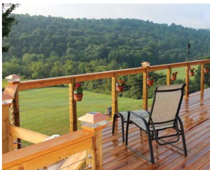
RailEasy™ Cable Railing (p.5) Customer supplied wood posts and handrails combined with 5/32" cable and tensioners as infill.
