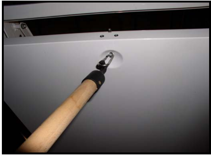
Pull door open using pole and hook.
