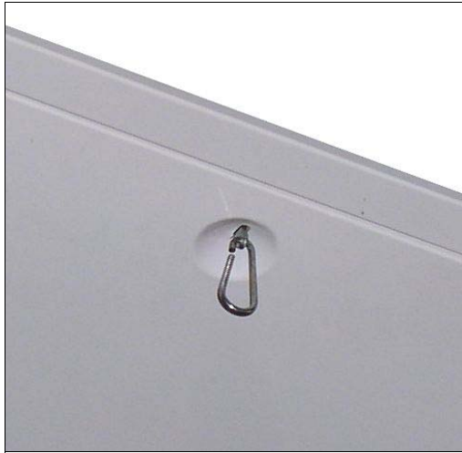
Slide door opening ring onto pin.
